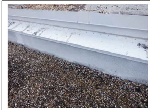
Expansion Joint at Walls to Roofs 2 & 3
