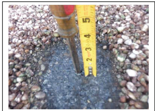
Roof 1 Core Depth at High Point (8" Total)
