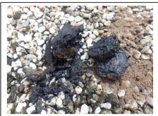
Roof 6 Core Cut
