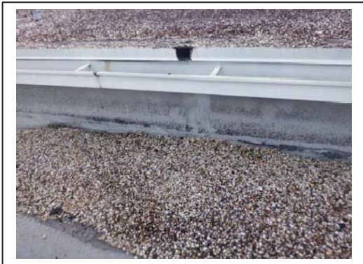
Base Flashing under Roof 1 Gutter and Drip Edge
