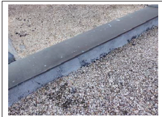
Expansion Joint between Roofs 1 and 2
