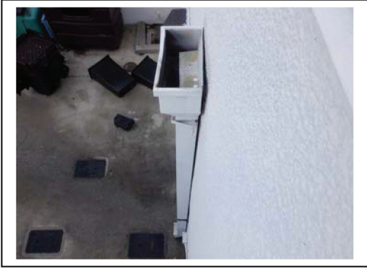
Leaderhead and Downspout
