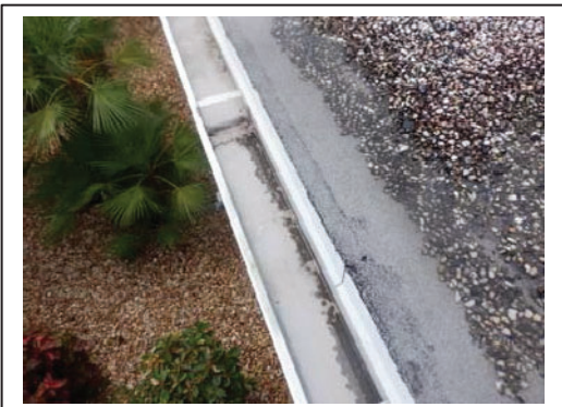
Drip Edge and Gutter
