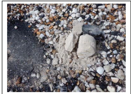
Roof 2 Core Cut
