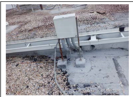
Conduit and Panel Stands in Pitch Pans
