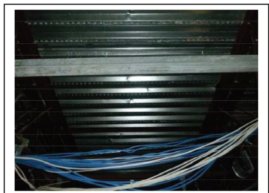
Underside of Roof 2 Deck
