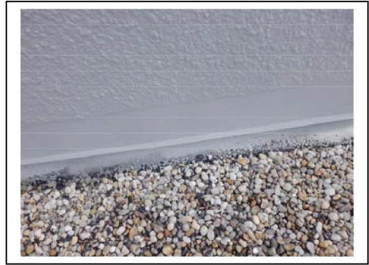
Base Flashing and Stucco Stop on High Wall
