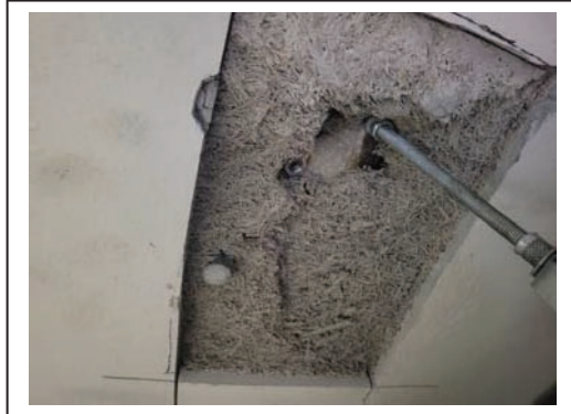
Tectum under Structural Concrete Deck
