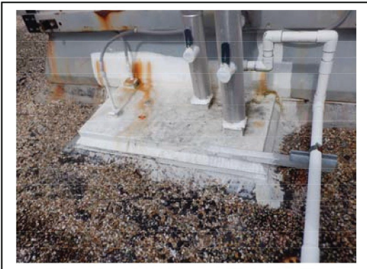
Pipe and Conduit Penetrations on Curb
