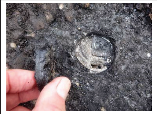
Roof 4 Core Cut to LWC
